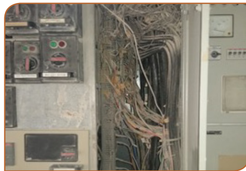
Images: Typical MCCs before (above) and after (below) an upgrade.
