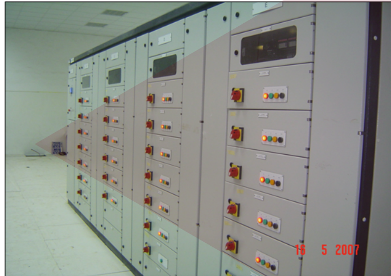
Compartment Back to Back MCC Panels
