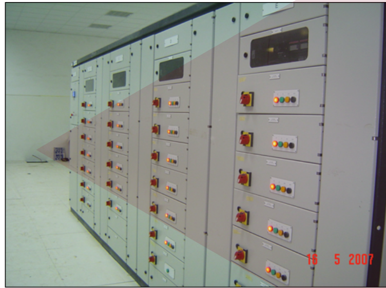
Compartment Back to Back MCC Panels
