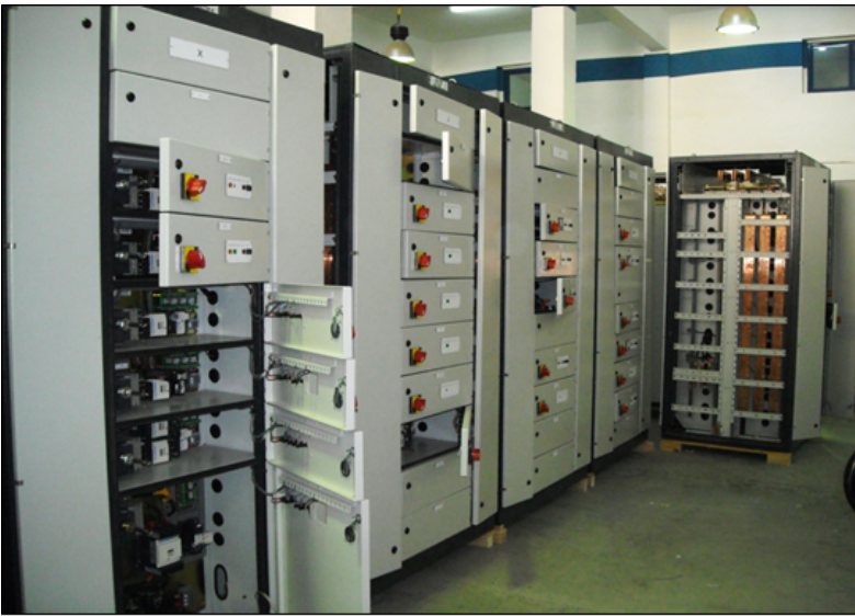
Compartment Back to Back MCC Panels
